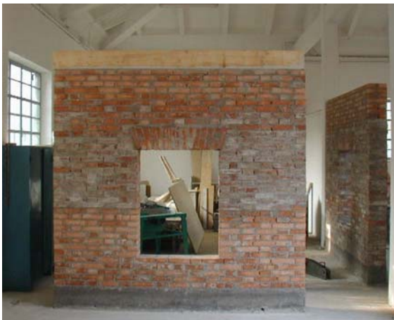
Fig. 3 Test perforated wall; texture 1
