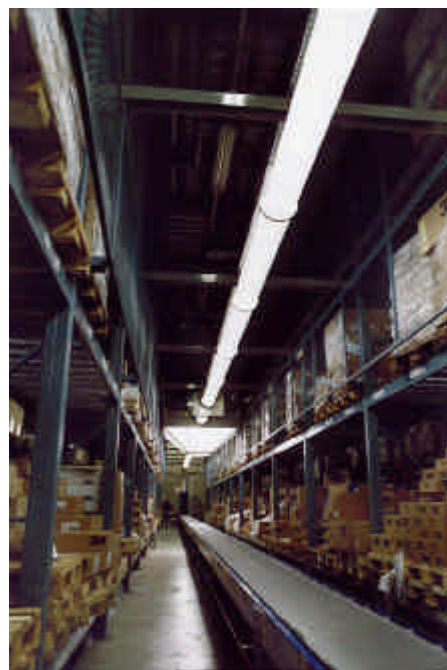
fig. 13: Coupling unit with hollow light guides.
